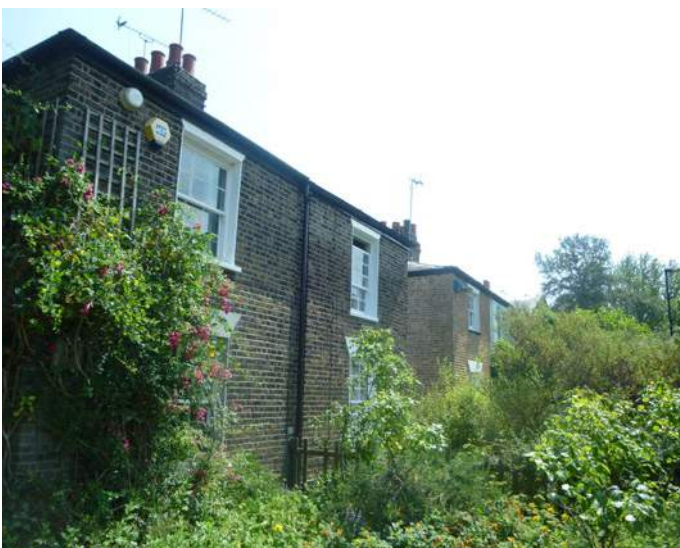
Prospect Place - Grade II listed cottages
