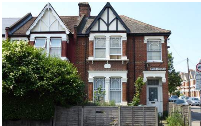
Bruce Grove: right-hand house with original sash windows; left-hand house with replaced windows and painted brickwork
