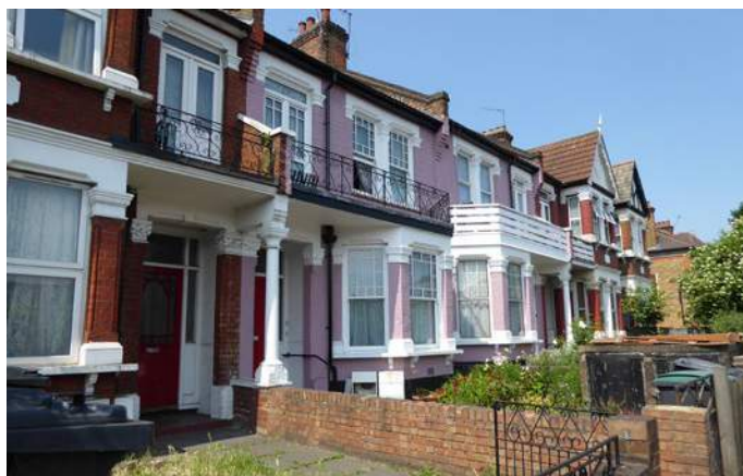
Bruce Grove: painting of brickwork
