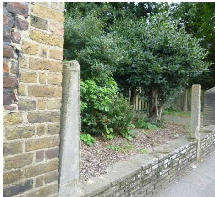
Church Lane – poorly integrated 20th century boundary walls to Bruce Castle
