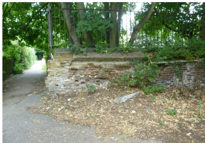
All Hallows Churchyard – north boundary wall in poor condition
