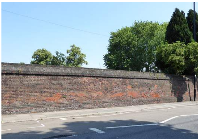
Lordship Lane: 17th century boundary wall to Bruce Castle Park
