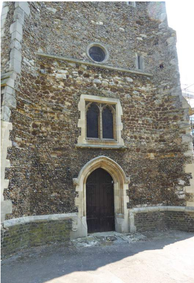
All Hallows Church tower – contrasting medieval building materials
