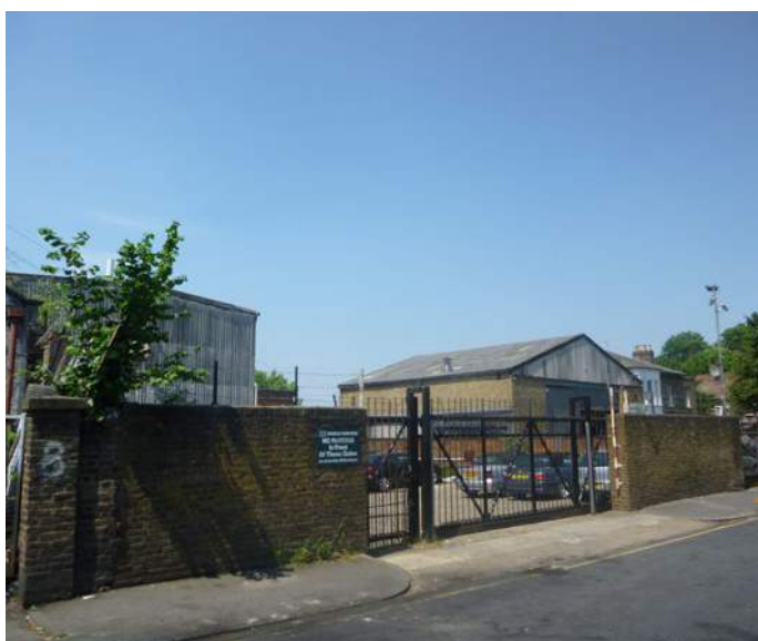
Church Lane – garages
