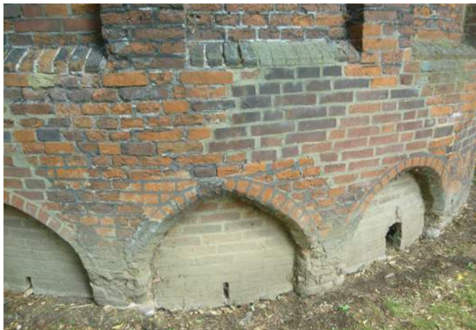
Bruce Castle tower – poor quality brickwork repairs and repointing
